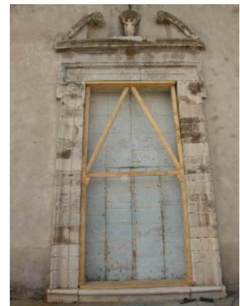
Figure 10.8: Propping and bracing door and window openings (SSN-DPC, 2005)
