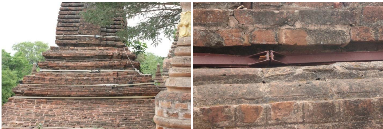
Figure 12.96: Monitoring time to time if tautness of synthetic belts and metal straps used for tying and confinement
