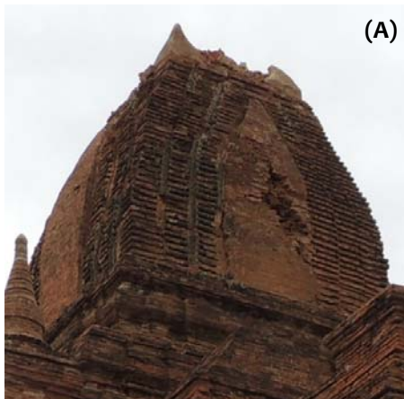
Figure 3.3: (A) Shear damage to the base of the spire; (B) Detachment and overturning of the free-standing pediment
