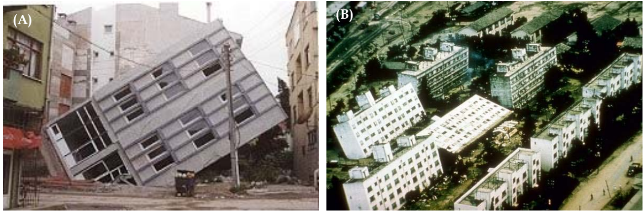
Figure 11: (A) Tilting of building due to liquefaction in the Kocaeli earthquake of August 1999; (B) Tilting of buildings due to liquefaction in the Nigata earthquake Japan, 1964
