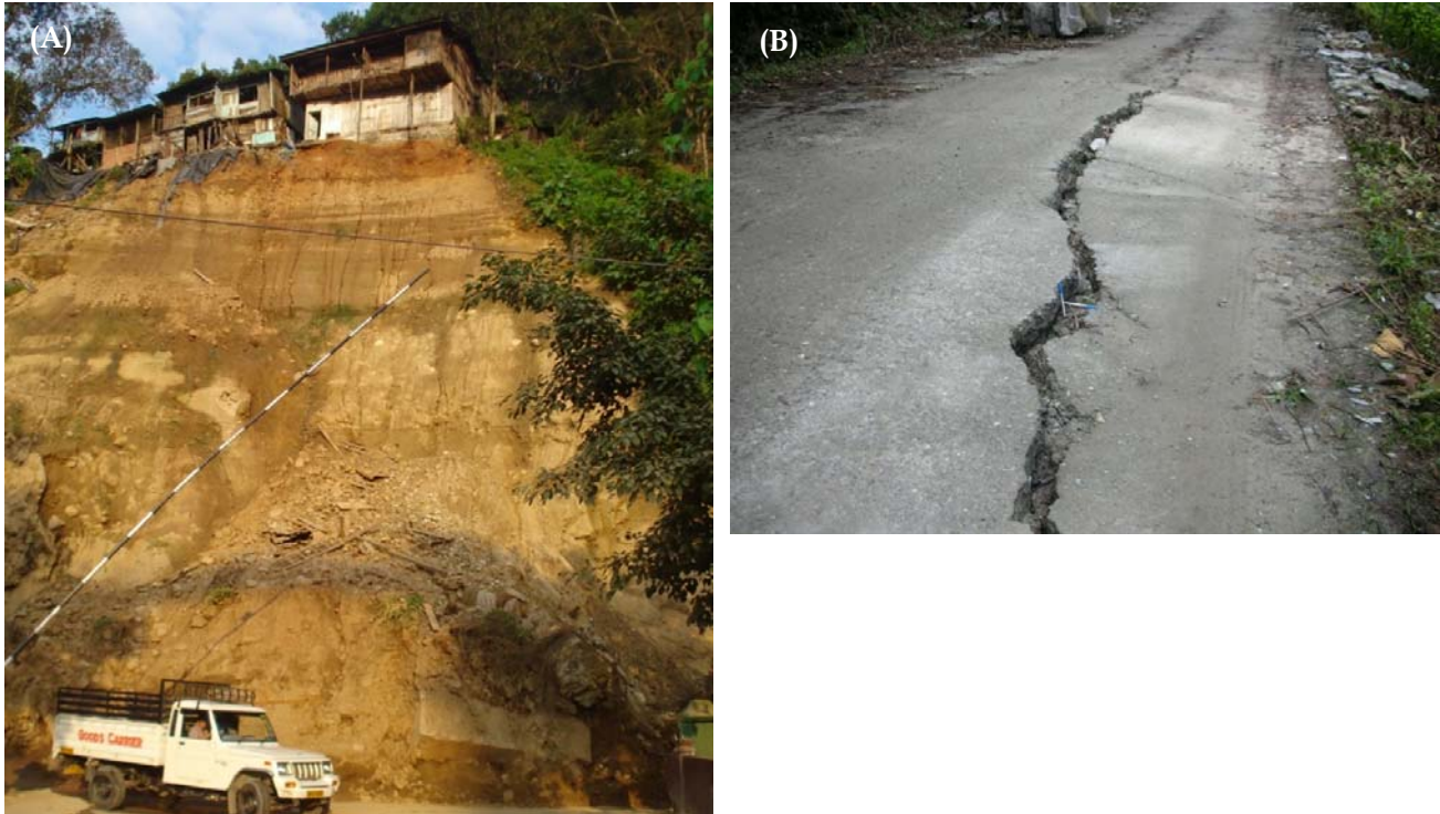
Figure 26: (A) Buildings precariously placed in landslide affected areas; (B) Ground fissures due to loss of slope stability in hill slopes or surface rupture due to fault movement
