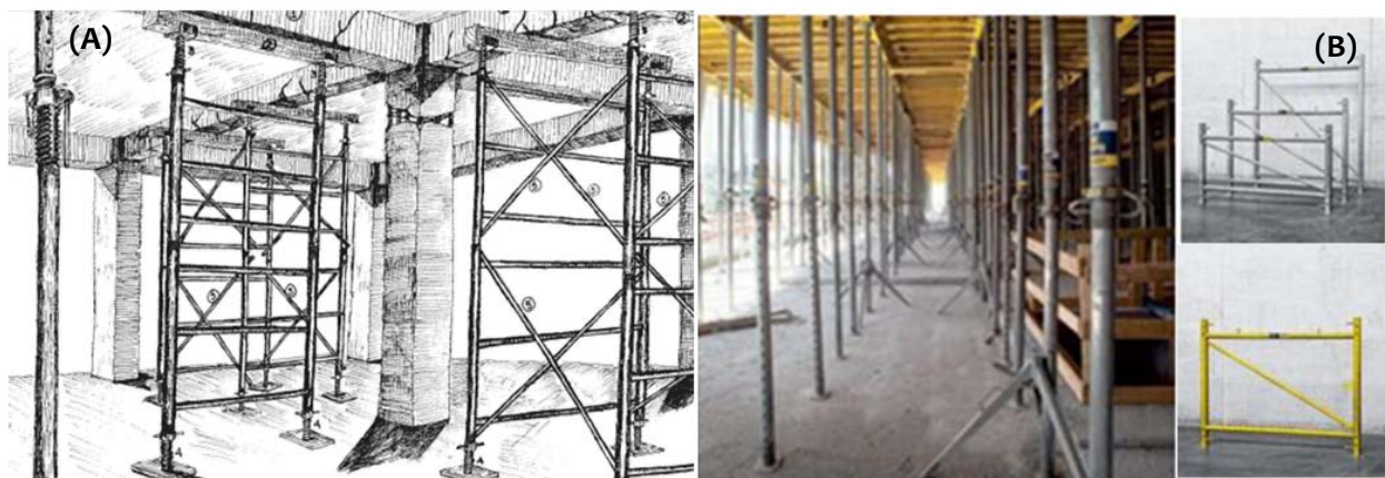
Figure 10.2: (A) Propping using Metal Industrial Scaffold (EPPO, 2000); (B) Larsen and Toubro's Doka Formwork System
