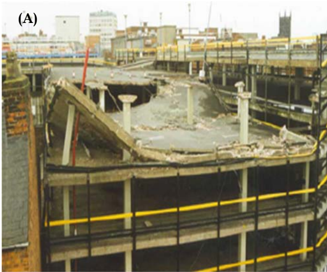
Figure 37: (A) Building showing punching shear failure in the flat slab; (B) Formation of punching shear damage at the interface of column and flat slab
