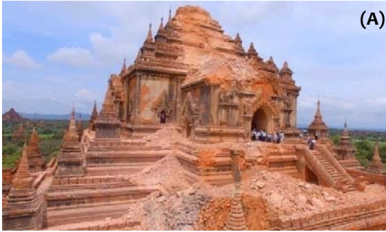
Figure 3.1: Collapse of spire
