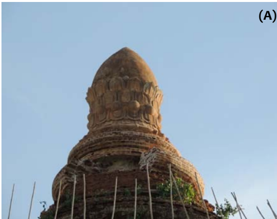
Figure 3.2: (A) Crushing of masonry due to flexural rocking at the base of the pinnacle; (B) Shear sliding of the pinnacle of the spire
