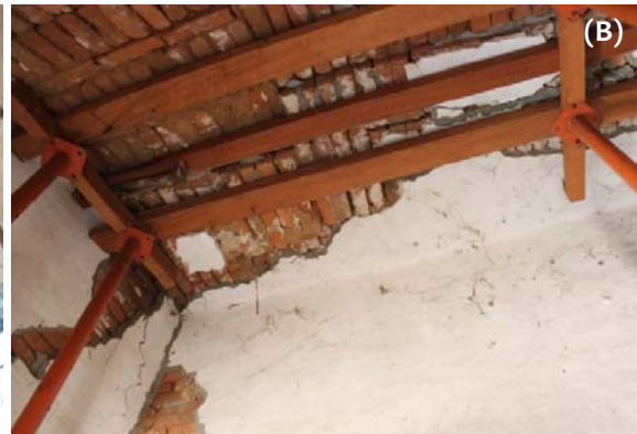
Figure 3.7: (A) Damage to vault due to dilation of masonry walls; (B) Deformation of brick masonry vault and dislodgement of bricks
