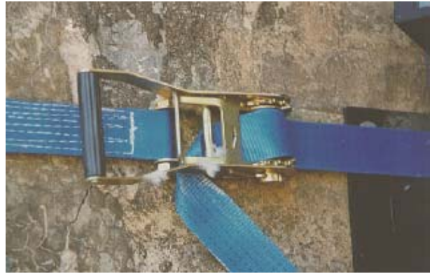
Figure 10.18: (A) Ratchet lashing to connect orthogonal walls (Langenbach, 2003); (B) Lashing and buckle
