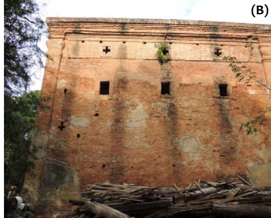
4. Figure 3.6: (A) Detachment and overturning of the facade; (B) Dilation of masonry walls and formation of vertical cracks
