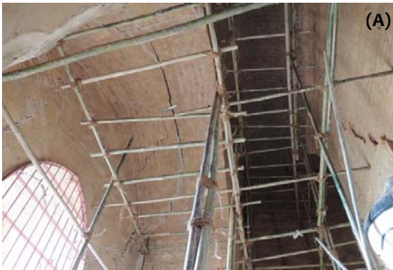
Figure 3.7: (A) Damage to vault due to dilation of masonry walls; (B) Deformation of brick masonry vault and dislodgement of bricks
