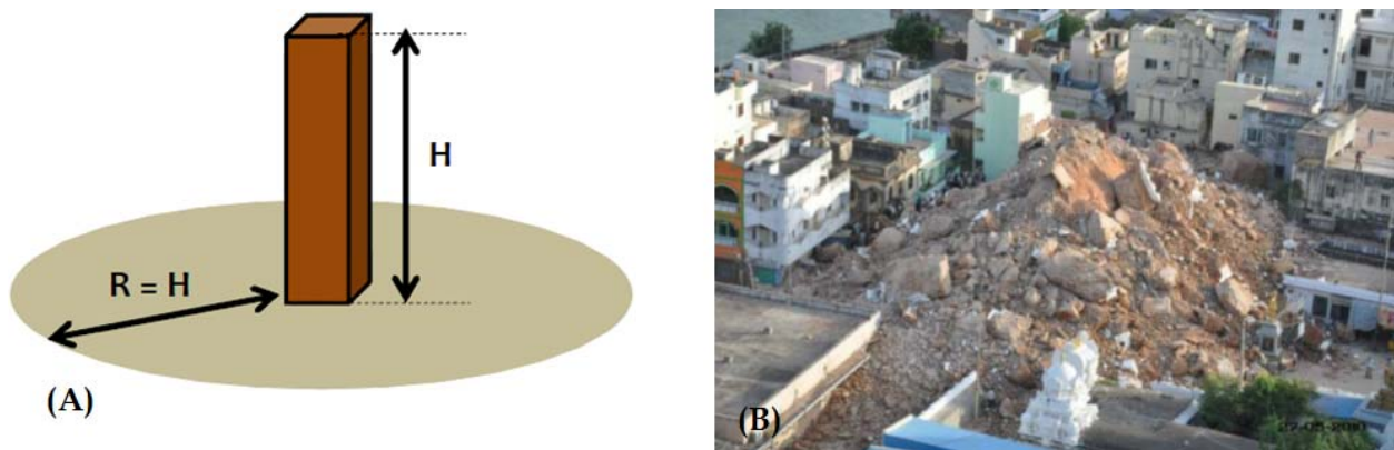
Figure 6.3: (A) Circular Area with Radius Equal to Height of the Structure to be Cordoned off (B) 7-Storeyed Temple tower collapse in Srikalahasti, India
