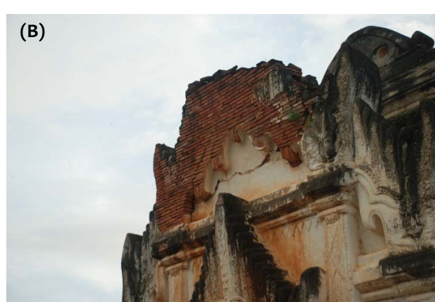
Figure 3.3: (A) Shear damage to the base of the spire; (B) Detachment and overturning of the free-standing pediment
