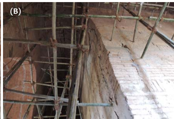
Figure 3.8: (A) Deformation of brick masonry vault and dislodgement of bricks; (B) Bulging and cracking in the solid core supporting the central spire
