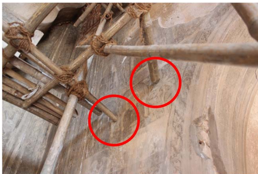
Figure 12.3: Ends of wooden structural members of the temporary stabilisation in direct contact with a wall with an ancient mural painting in Bagan
