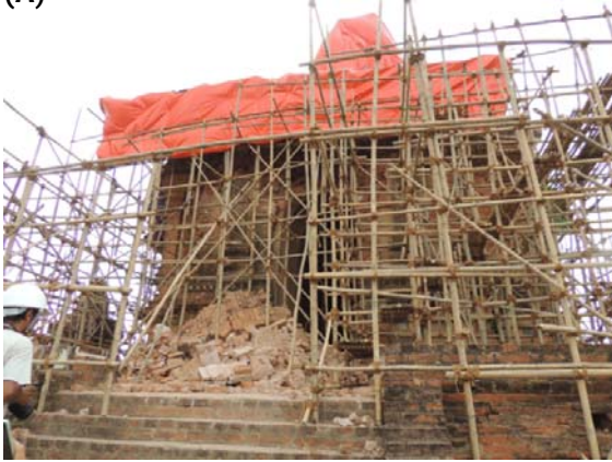
4. Figure 3.6: (A) Detachment and overturning of the facade; (B) Dilation of masonry walls and formation of vertical cracks
