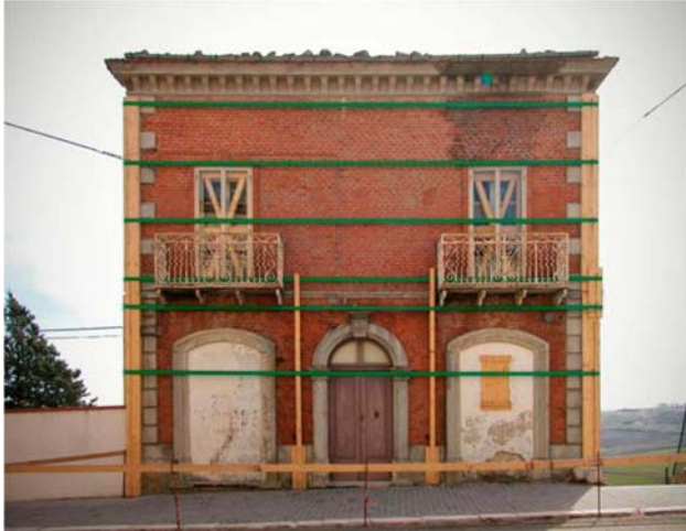
Figure 10.18: (A) Ratchet lashing to connect orthogonal walls (Langenbach, 2003); (B) Lashing and buckle
