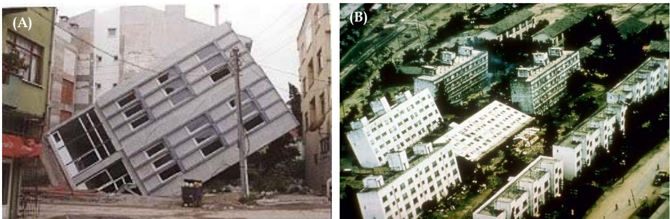
Figure 27: (A) Tilting of building due to liquefaction in the Kocaeli earthquake of August 1999; (B) Tilting of buildings due to liquefaction in the Niigata earthquake Japan, 1964
