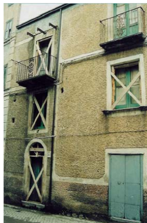
Figure 10.8: Propping and bracing door and window openings (SSN-DPC, 2005)
