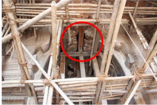
Figure 12.85: Congested temporary intervention
