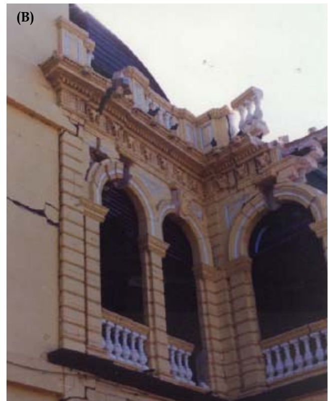
Figure 22: Dislocation and collapse of the keystone (at the crown) and voisseurs (other units) of the arch
