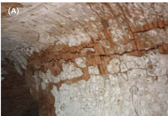
Figure 3.8: (A) Deformation of brick masonry vault and dislodgement of bricks; (B) Bulging and cracking in the solid core supporting the central spire
