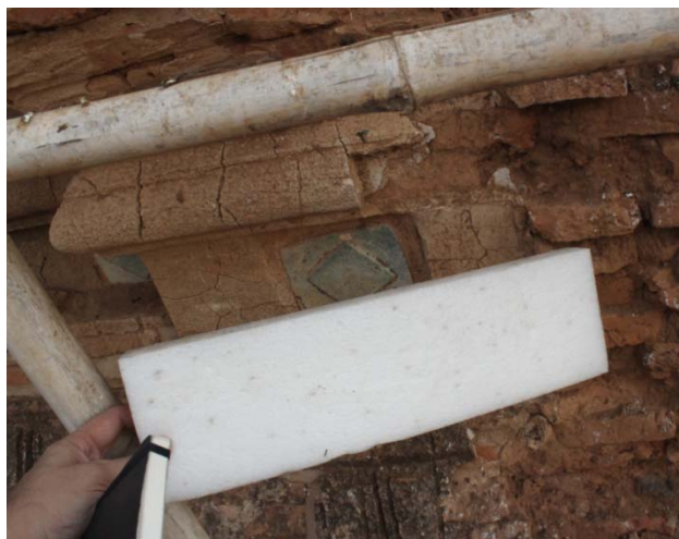
Figure 12.52: Introduction of EPE foam sheet over the niche with the glazed tile
